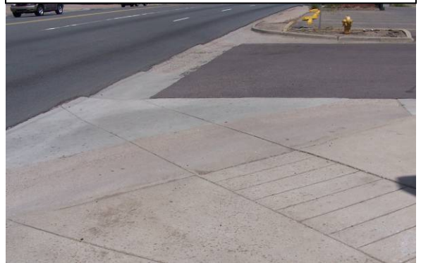
Non-ADA curb ramp at southeast corner of 10th Avenue/Wadsworth Boulevard
