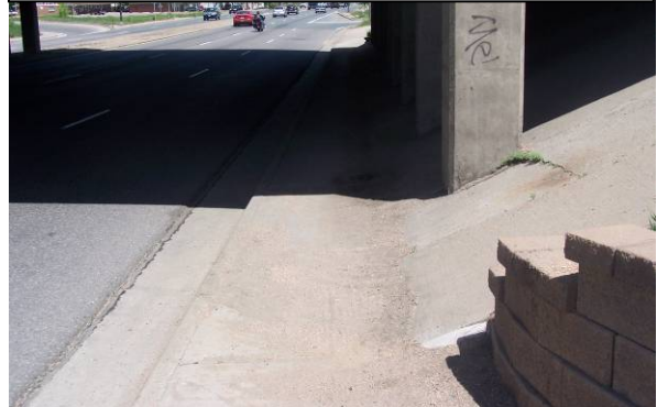
Missing curb ramp on northeast corner of 8th Place and Wadsworth
