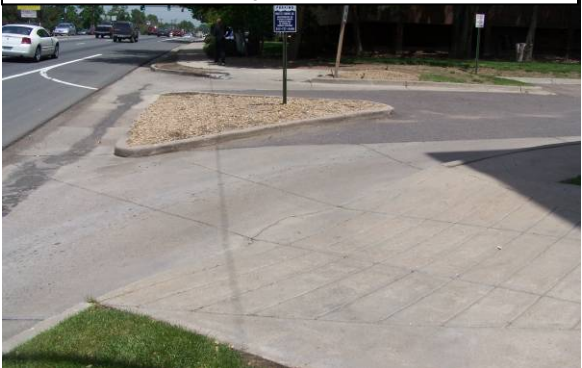
Turn island without curb ramps in pedestrian path (940 Wadsworth Parking Lot Access)
