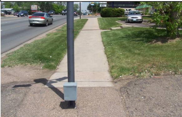
Turn island without curb ramps in pedestrian path (940 Wadsworth Parking Lot Access)
